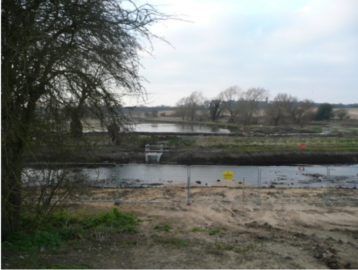
1. Aldhurst Farm: newly constructed ponds. (R. Fulcher, 2015.)
